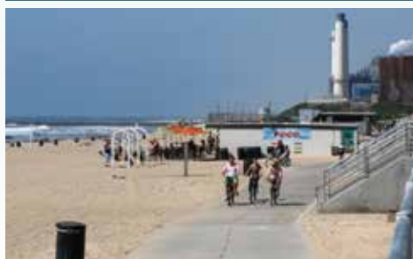
Permeable Concrete Path
