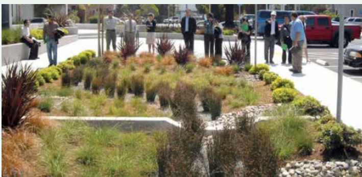
Bioretention Internal Weir
