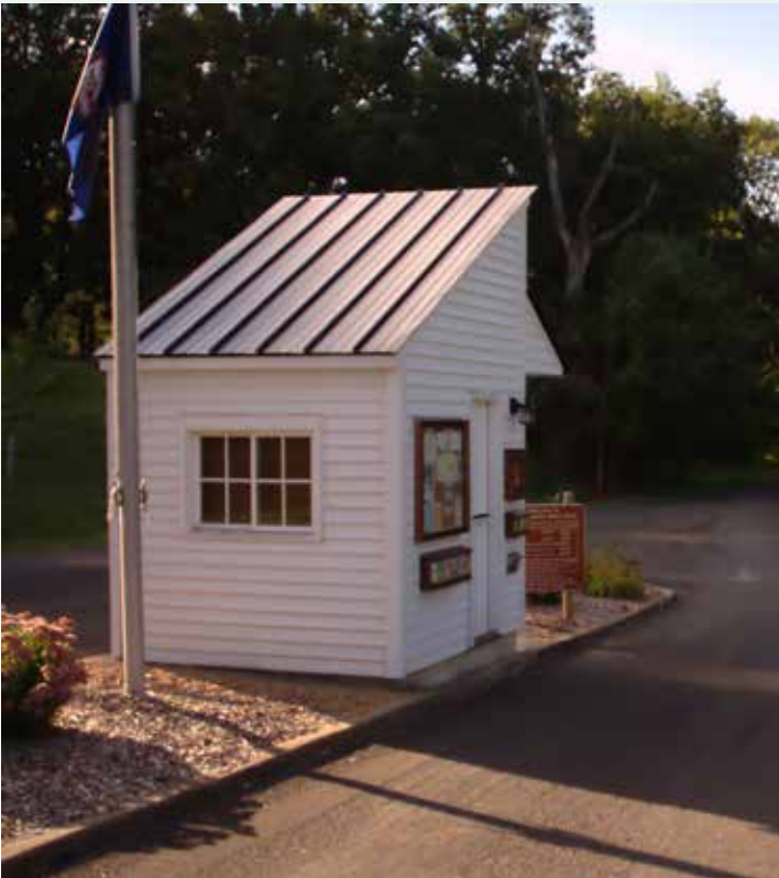
Stick-built Station with White Clapboards
