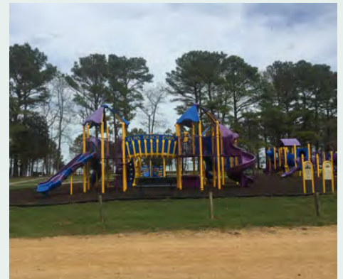
Existing play equipment
