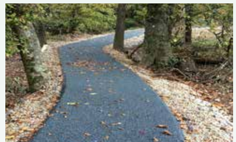
Permeable Flexible Pavement
