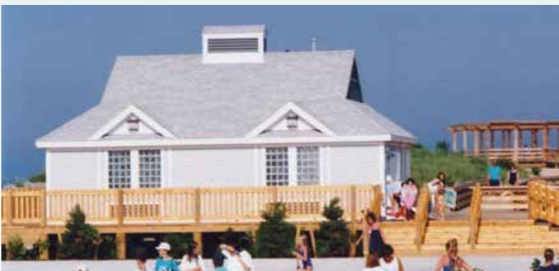
Beach Composting Comfort Station & ADA Accessible Ramp
