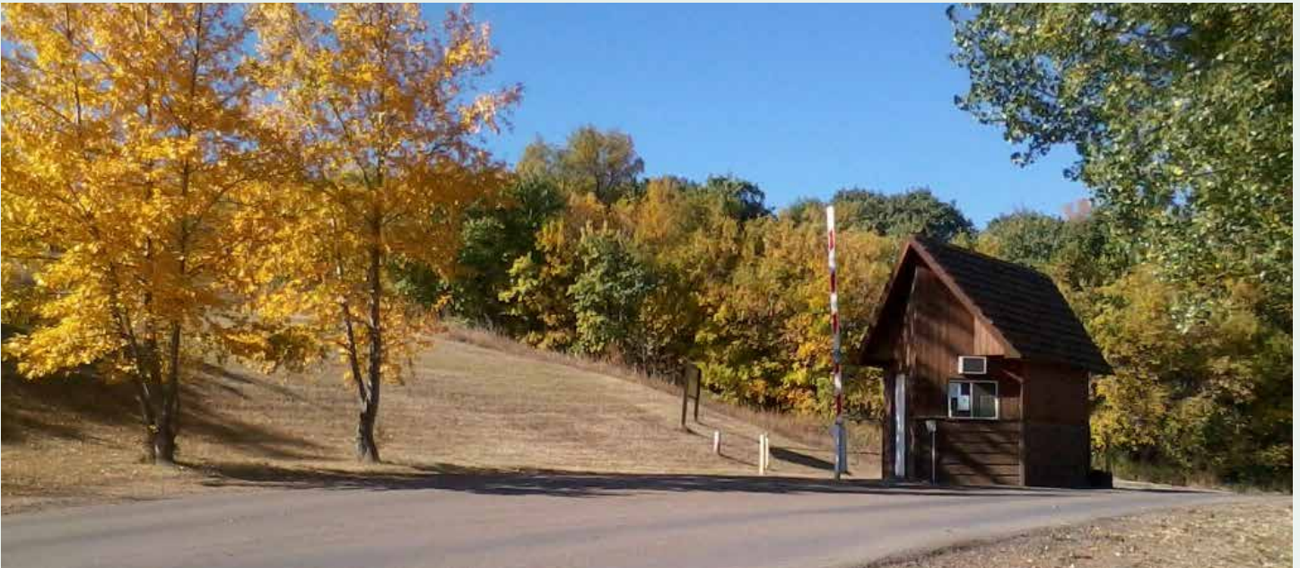
Prefabricated Station with Board & Batten Concrete Form-liner
