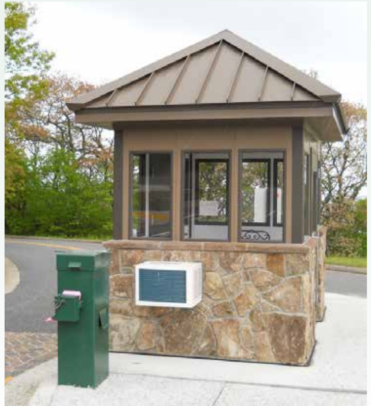
Prefabricated Station with Stone Embellishment
