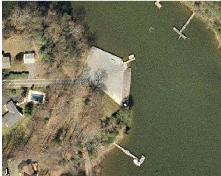
Forest Landing, shown above, before improvements were made.
