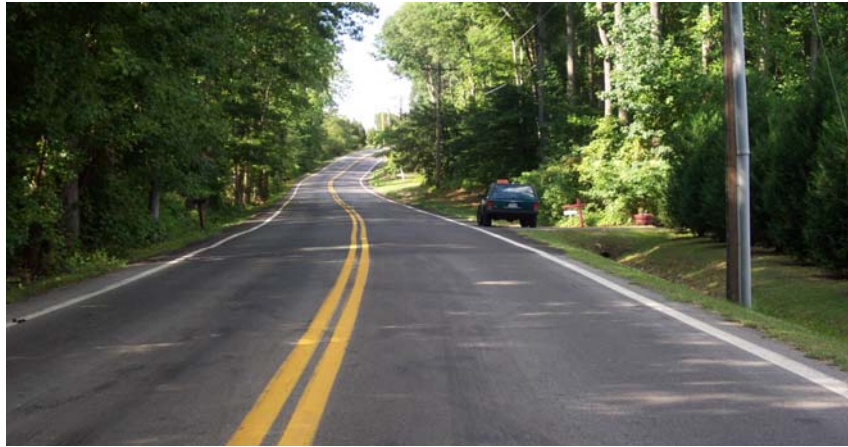
MD 236 is a high speed/moderate volume collector roadway frequently used by carriages although there are limited shoulders throughout most of the roadway.
